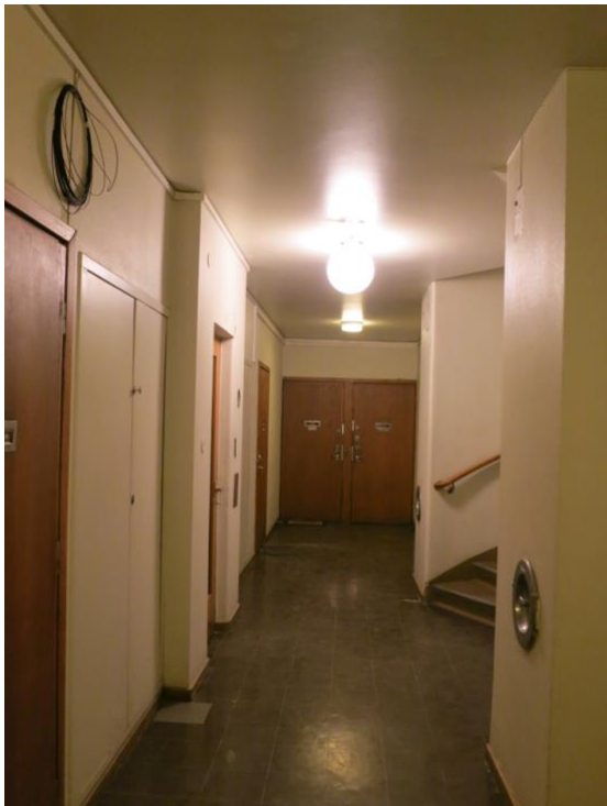
Test luminaire, round globe is tested in front of the lift. Further away, a round, flat one from the 1970s still sits. New cable strip installed at the ceiling and the fiber runs have begun.
