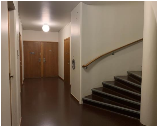
The entrance doors have been surface-renovated by cleaning and oiling/waxing. All fittings have been retained, signage is kept uniform according to brf's rules.
