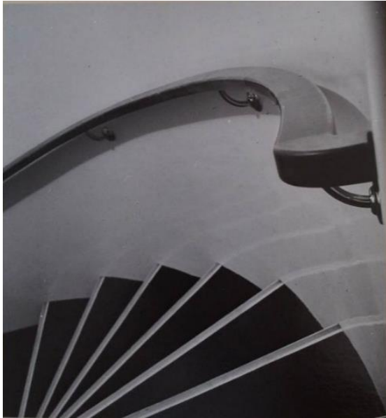
Original staircase, 1935. NOTE no painted plinth against the wall, according to drawing.
