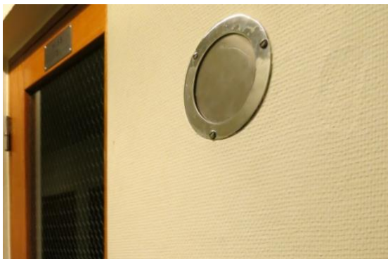
New number is proposed to be painted on blasted glass in the round hatch with weak lighting behind.
