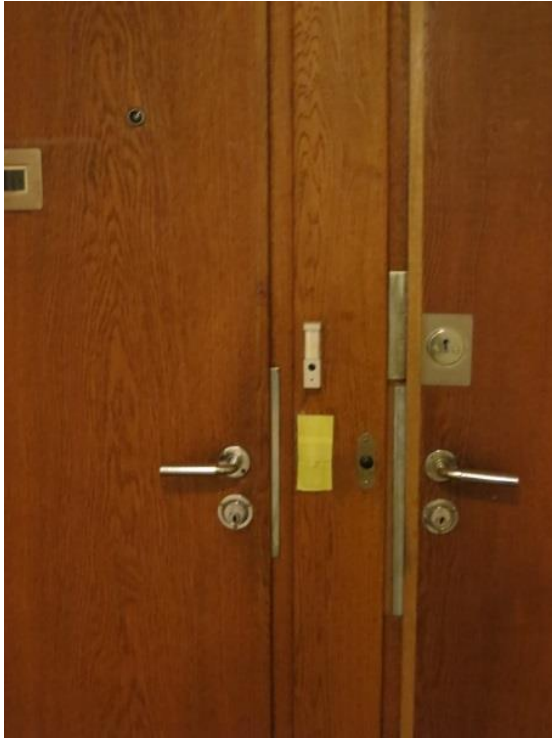
Adjustment and overhaul of all door fittings is carried out before painting.
