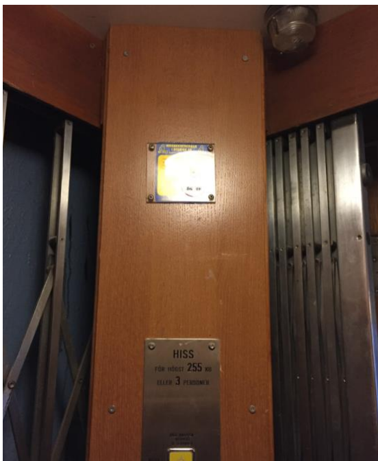
In connection with the replacement of the lift slab, restoration to the original edge detail on the diagonally placed board is discussed.
