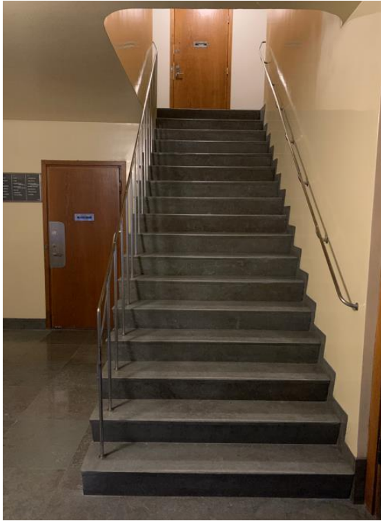
The limestone stairs have been cleaned of non-slip tape and polish and small damages, e.g. on the exposed outer corner of the lower step, have been repaired with stone repair cement.
