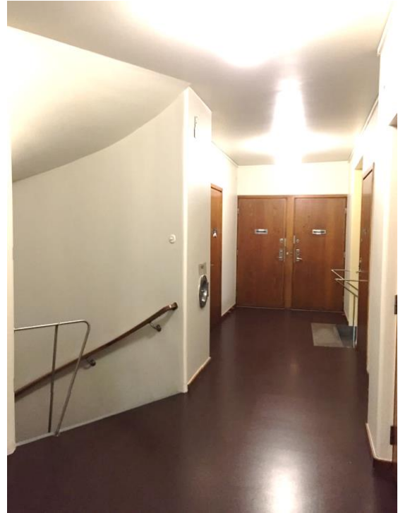
New stair railing to protect against falling down the basement stairs on the left. Design inspired by the main staircase in the foundation and below, design AIX Arkitekter.
