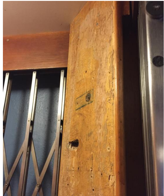
The original design with rounded edges emerged during disassembly but was badly damaged.
