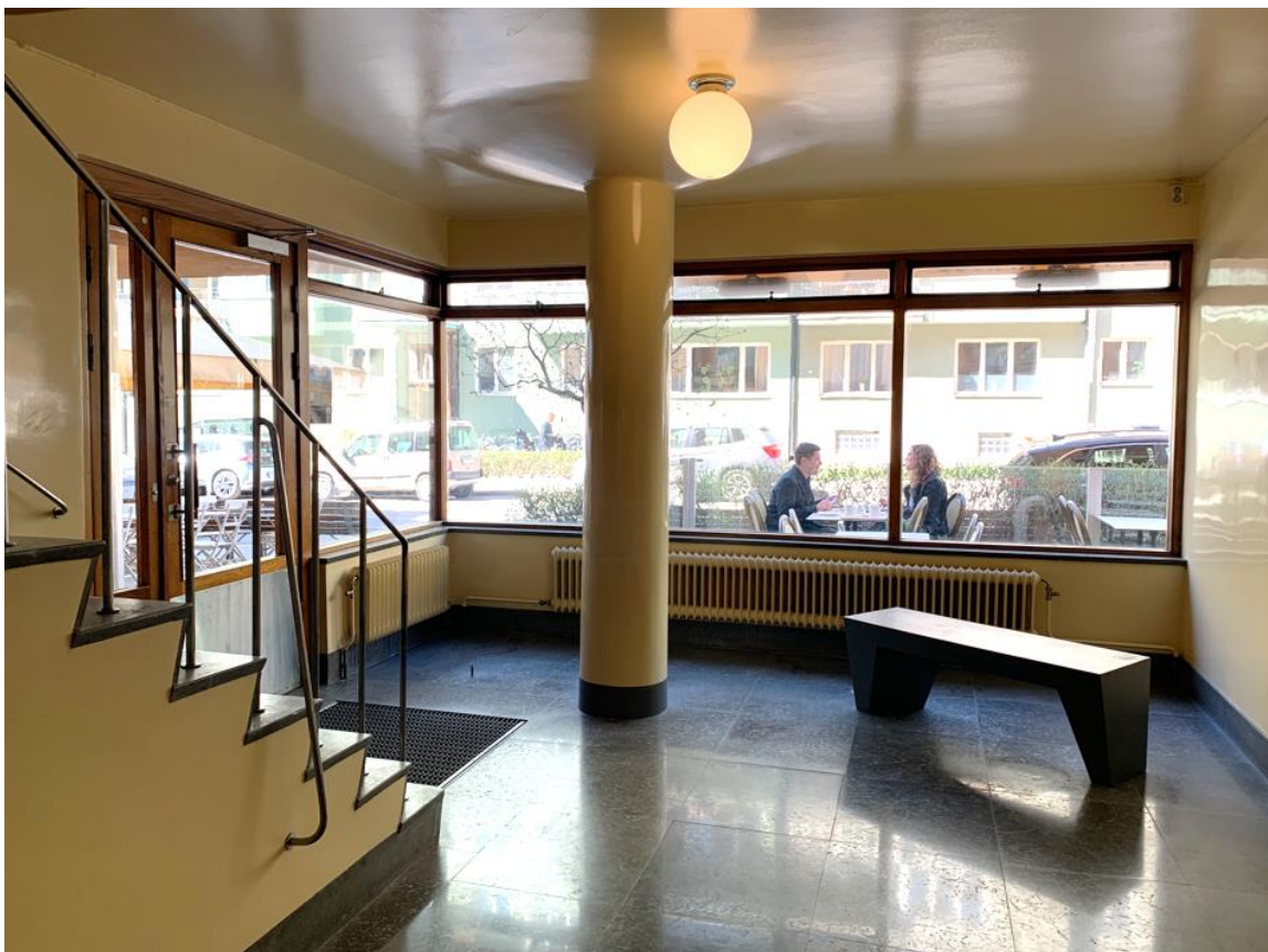
The floor of the entrance vestibule has regained the varying colors of the limestone after removing many layers of yellowed polish.
