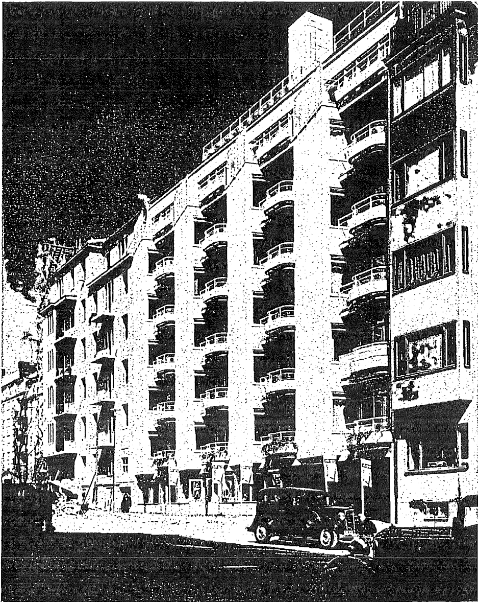
The street façade. The cantilevered walls, besides giving interest to the elevation, serve to screen each balcony from its neighbour.
