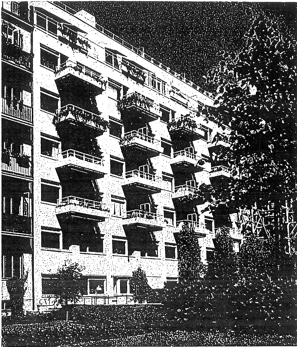
The rear elevation, showing the large balconies which virtually constitute an additional room.
